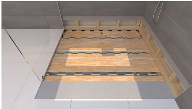
3. Recess Recess the subfloor.
